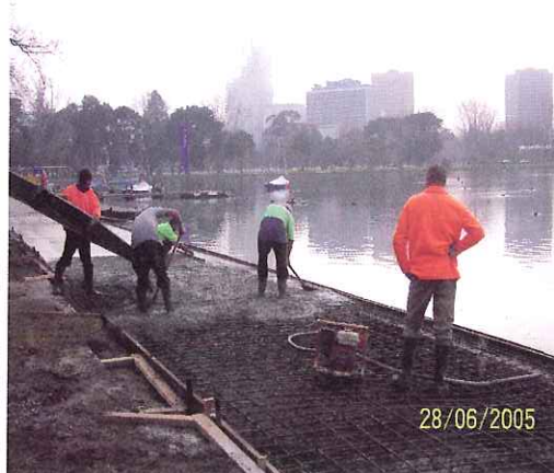
Heavily Reinforced Concrete Walkway
