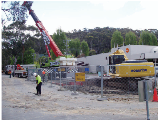
Road Reserve, Tank Installation
