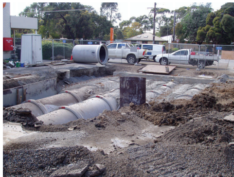
Storage Tank, In Ground
