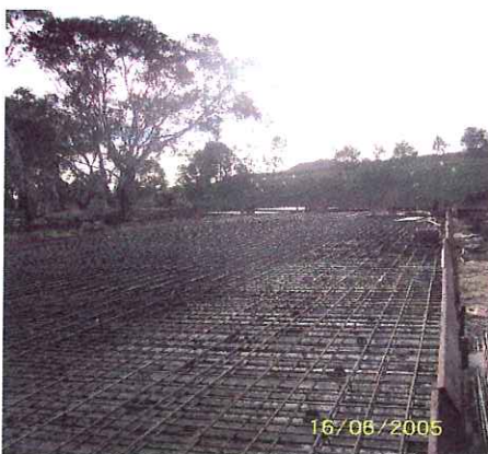
Heavily reinforced cover slab
