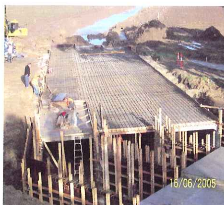
Insitu transition structure between culverts
