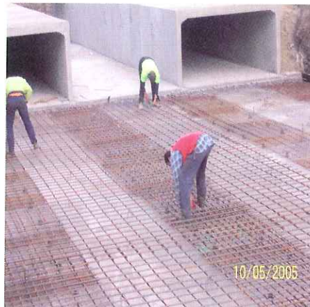
Steel fixing for culvert slabs
