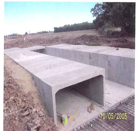
Box culverts installed prior to cover slab
