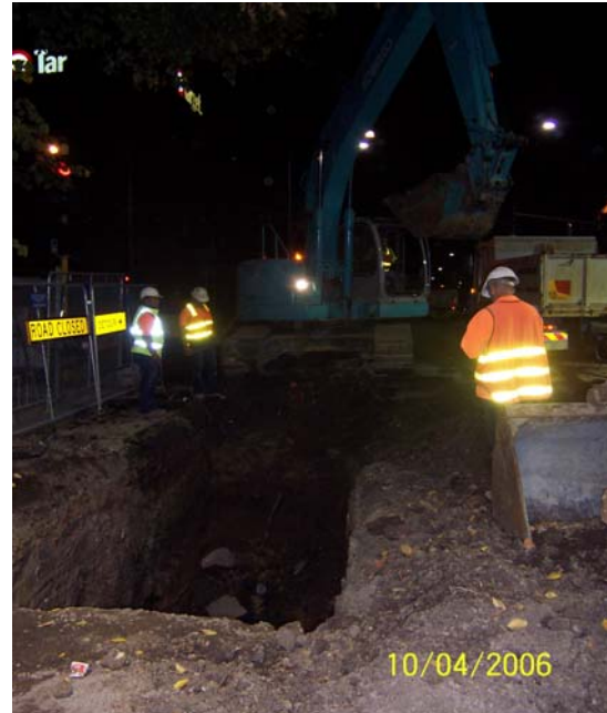
Locating Services in Brougham Street
