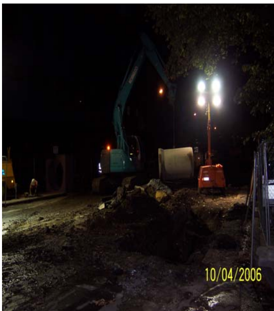
1350 dia RCP Installation
