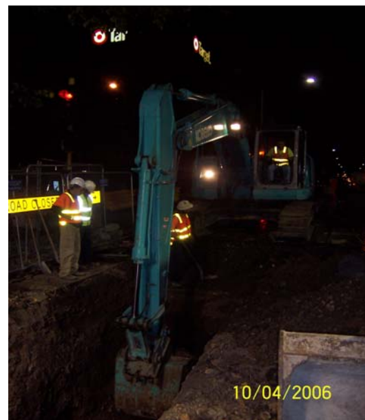
Pipe Line Excavation
