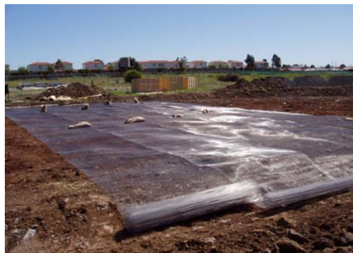
Placement of Stainless Steel Mesh
