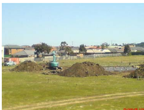
View towards Excavation Works
