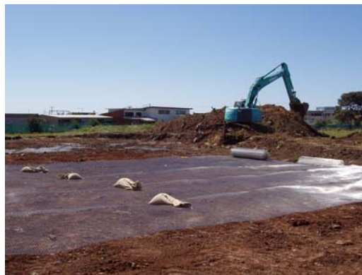
Excavation for Placement of Stainless Steel
