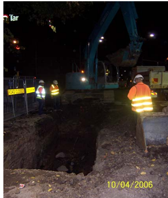
Locating Services in Brougham Street
