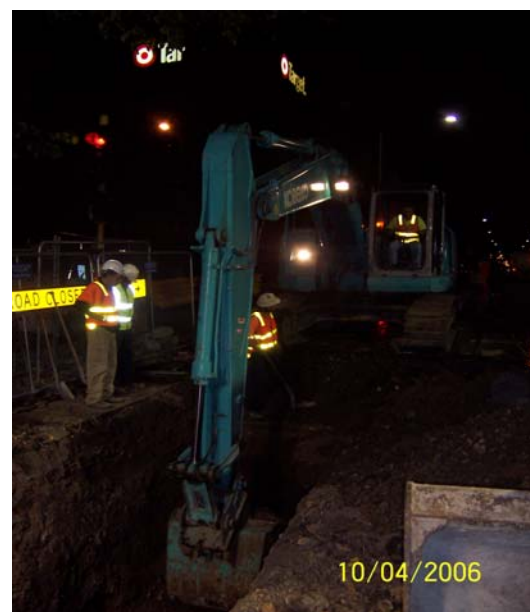
Pipe Line Excavation
