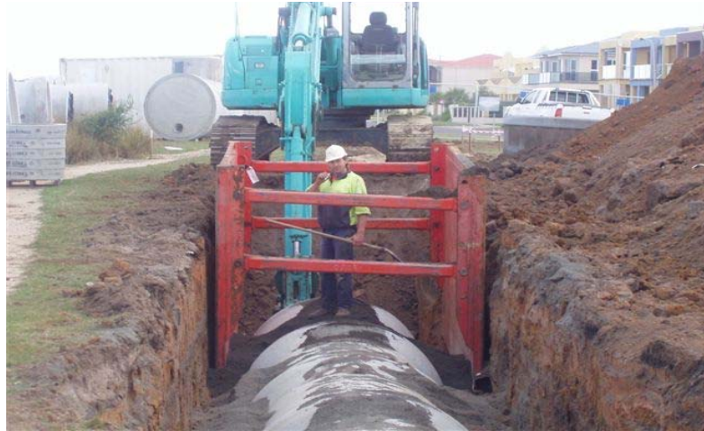
Plastiline Sewer Main Installation
