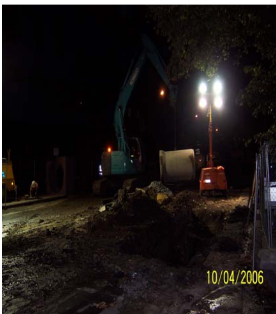
1350 dia RCP Installation
