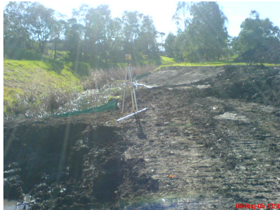
Shaping of Creek
