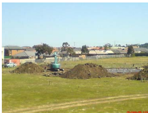
View towards Excavation Works
