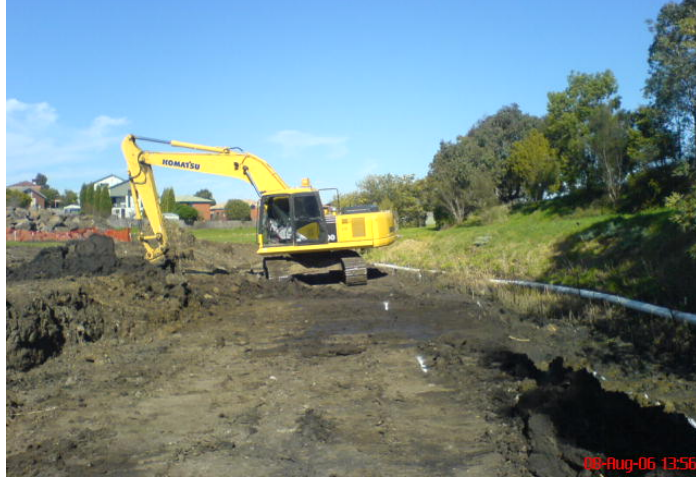
Excavation of Creek Bed
