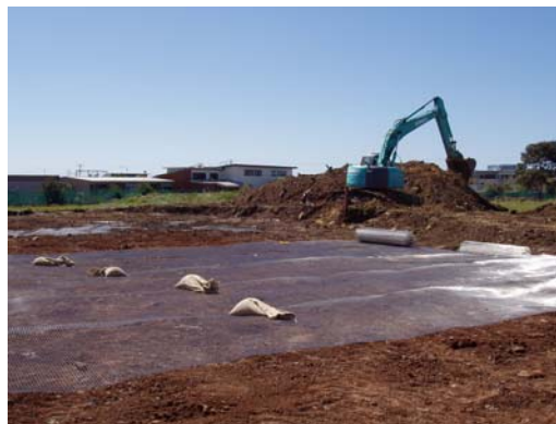
Excavation for Placement of Stainless Steel
