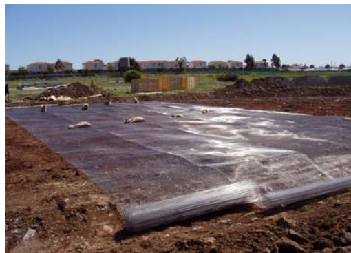
Placement of Stainless Steel Mesh
