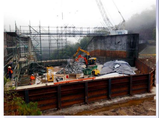
Clarrie Hall Dam is a rock-filled embankment dam located on Doon Doon Creek, a tributary of the Tweed River, approximately 4 km south west of Uki. The 15,000 ML litre reservoir provides the drinking water for the Tweed Region. Tweed Council is upgrading the Spillway to meet the Dam Safety Committee's Requirements and to ensure that the dam can continue to safely pass extreme flood events.
